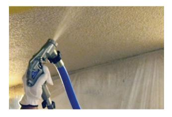
The objective is to spray and trowel the basecoat onto the Even Better Acoustical Board at 3 mm (1/8") wet thickness as the dry thickness will be approx. 1.5 mm (1/16").
