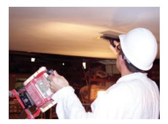
Have third applicator make a final pass over the Even Better 2 plaster within 15–20 minutes of the initial application, using the flexible finishing trowel.
