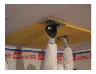
Slot the Even Better Acoustical Board into the C channel without exerting any significant pressure and use the Fellert Trowel to steady the board as you position it correctly.
