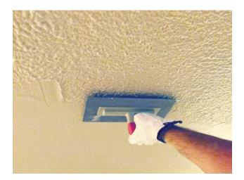
Spray a, as thin as possible, layer of the Even Better 2 Silk plaster on to the surface and trowel as smooth as possible. Do not over trowel the plaster. Have two applicators troweling the Silk plaster smooth immediately upon spraying. Closing in the surface and removing the excess plaster. As the plaster takes up (surface moisture decreases) you may need 2-3 separate passes with the trowel over the surface in order to achieve a consistent finish, approx. 4-5 minute in between passes.
