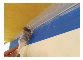
Apply the 50 mm (2") self-adhesive mesh tape to bridge the plastic C channel, plastic trims, drywall rippers and board transitions to other substrates.
