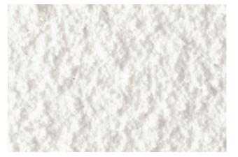
Spray consistently and eliminate spattering on plaster surface. Leave to dry 1-2 days.
