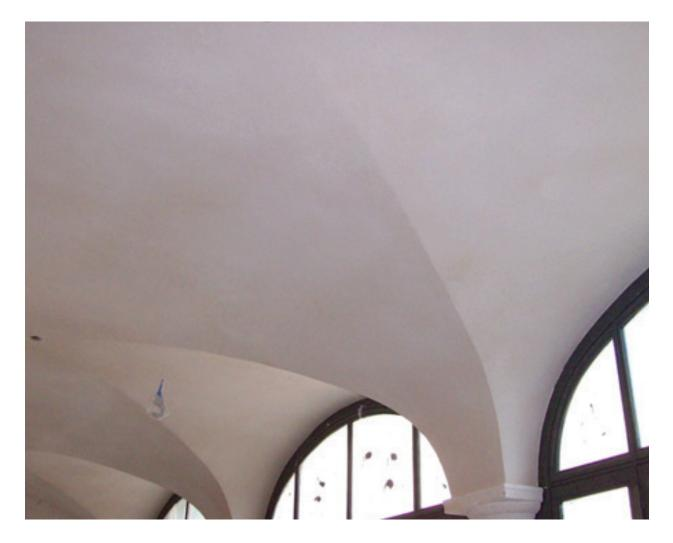
Installation of curved surfaces is to be done with the adhered to GWB method.
