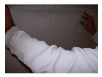
Apply approximately 30% of the basecoat as normal to the surface. Place each vertical length of mesh as you proceed along the length of a wall spraying basecoat. Do not overlap the mesh. Try and butt the lengths as tight as possible. A small gap of 13 mm (1/2") is acceptable.
