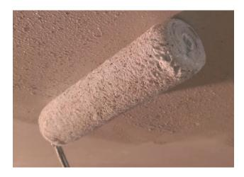
Apply the Even Better Primer mixed with Primer additive to the drywall substrate with a short nap roller.
