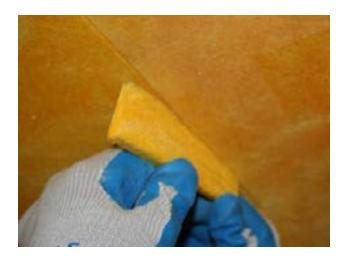
Remove masking tape when complete. Leave the Fellert Primer to dry overnight. Never apply Fellert Plaster and Primer the same day.
