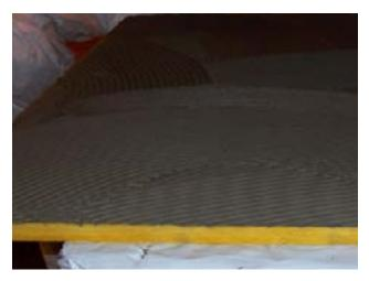
Wherever possible install the Fellert acoustical boards so the longest runs of joint lines flow into and away from the strongest source of light. This process is deemed a "best practice" only and not an absolute rule. It is a simple and a logical approach to help minimize any shadowing effects which can be exacerbate by critical lighting.
