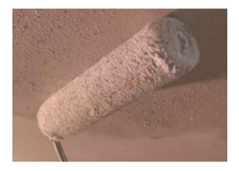
Apply the Fellert Primer to the drywall substrate with a short nap roller.
