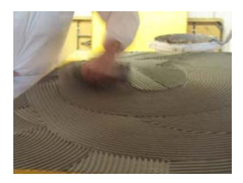
Finish off the adhesive application by straightening the 6 mm (¼") notched lines. This will ensure an even layer of adhesive on the drywall ceiling.
