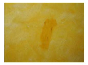
**Resin Spots:** Must be treated by cutting into the affected basecoat and Fellert Acoustical Board to remove the resin deposit. Fill the extracted area with new board, basecoat and sand when dry.
