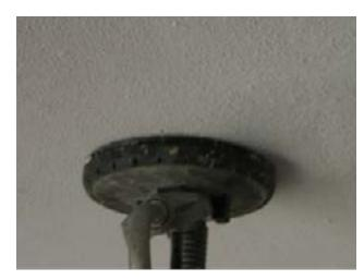
Pre-filling of any joints or variances in the basecoat is very important. Spot apply EB1 to any rippers, beads, board joints, etc. as needed and let dry. When dry, sand out any ridge lines or surface unevenness from the basecoat application. Sand the entire surface of the basecoat with 220 grade sanding discs.
