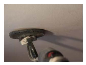
The Silk finish consists of a base layer of EB1 and a finish coat of EB2 plaster. Sand the base layer application with a 220 grit sanding disc and sanding sponges. Once sanding is complete all imperfections should be eliminated including any board joints, holes, or trim details.
