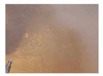
The objective is to spray the EB2 finish onto the basecoat leaving a fine sprayed texture, at 1.5 mm (1/16'') wet thickness.
