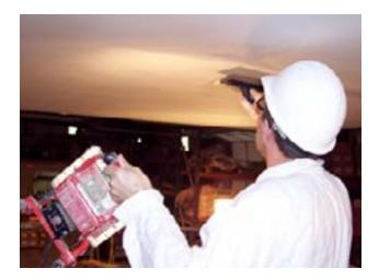
Have third applicator make a final pass over the EB2 Silk plaster within 15–20 minutes of the initial application.
