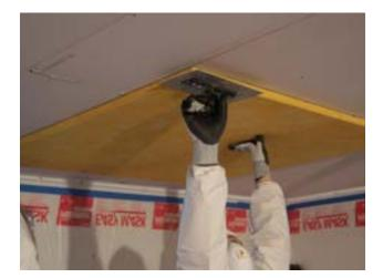
Slot the Fellert acoustical board into the C channel without exerting any significant pressure and use the Fellert Trowel to steady the board as you position it correctly.
