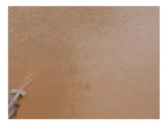
The material flow would normally be set the 3rd ascending dot on the Graco RTX 1500. Mix up the EB1 finish coat in the same manner as the basecoat.
