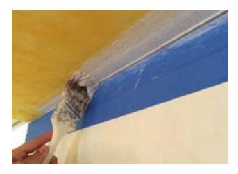
Apply the 50 mm (2") self-adhesive mesh tape to bridge the plastic C channel, plastic trims, drywall rippers and board transitions to other substrates.
