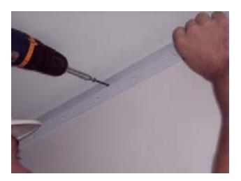
Screw the plastic C channel trim into the perimeter wall 400 mm c/c (16" o.c.) studding and not the ceiling.
