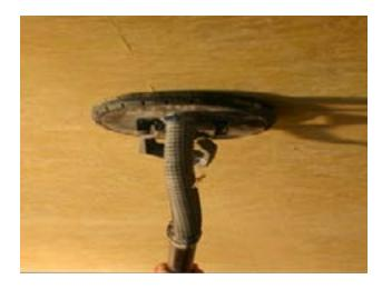
Sand the entire surface of the acoustical board in a gradual circular motion to ensure the board joints are sanded flush and all variances are sanded out, i.e. eliminating valleys, "low points or lines" in the board substrate. Use 80 grit full size sanding disc pads. The completed board installation should appear to be consistent with no variances in thickness. Ensure the critical lighting is in place prior to sanding to ensure any variances are sanded.
