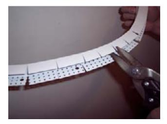
Use the straight-edged snippers to bend the plastic C channel around any curves and angles.
