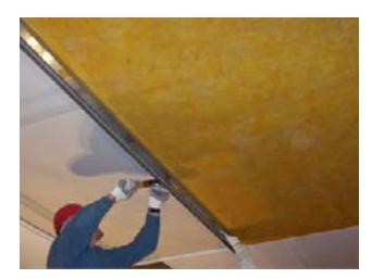
As you progress with the installation of the acoustical boards you may have to periodically "straighten the line" as depicted. The Fellert Acoustical Boards are manufactured to a tolerance of 3 mm (1/8"); therefore, this straightening process is normal.
