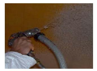
The objective is to spray and trowel the basecoat onto the Fellert Acoustical Board at 3 mm (1/8") wet thickness as the dry thickness will be approx. 1.5 mm (1/16").
