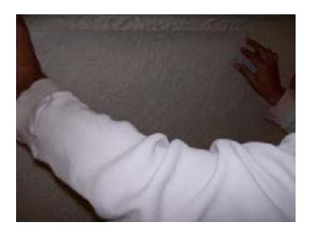
Apply approximately 70% of the basecoat as normal to the surface. Place each vertical length of mesh as you proceed along the length of a wall spraying basecoat. Do not overlap the mesh. Try and butt the lengths as tight as possible. A small gap of 1.3 cm (1/2") is acceptable.
