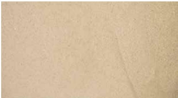
Try to eliminate all trowel lines and low-points on the surface.
