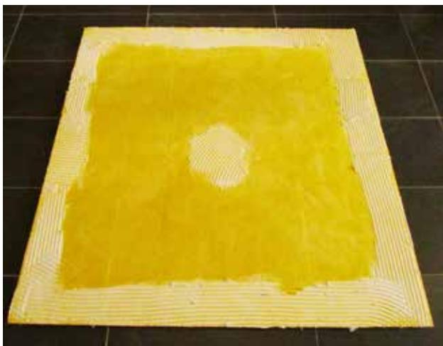
Apply the Even Better Adhesive to the back of the board by using a 6 x 6 mm or 1/4” notched trowel. Ensure to apply the adhesive along all edges of the board and at all ceiling penetration cut outs. Apply a few dots of glue in center of board as well. Press the board and shear it into place. (see picture to the left). Uneven or curved surfaces require more adhesive.
