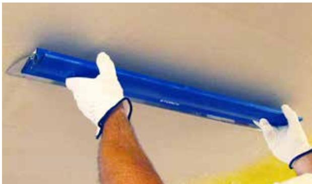
The more you trowel the more uneven the plaster surface becomes. Do not excessively trowel the basecoat plaster.
