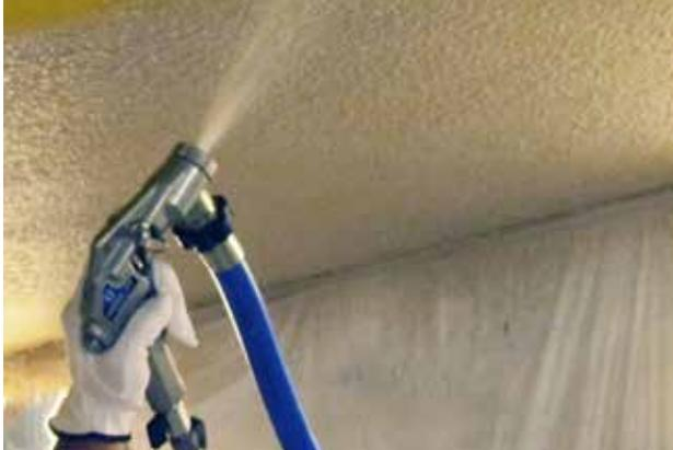
The objective is to spray and trowel the basecoat onto the Even Better Acoustical Board at 3 mm (1/8”) wet thickness as the dry thickness will be approx. 1.5 mm (1/16”). 3 mm(1/8”) thickness corresponds to just thick enough to eliminate yellow shine through from the board. Tip Size: Graco - size 10 - pressure at 4.5 to 5 dots Inomat M8 - size 8 or 10
