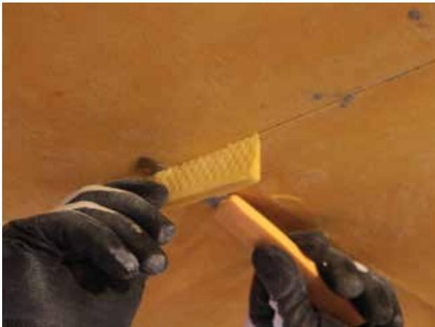
Ensure the spliced material is wedged very tightly into any gap and cut flush in preparation for sanding. You can use the beveled cut shavings from the boards that were inserted into the C channel. It is critical that the boards are installed and prepped correctly.
