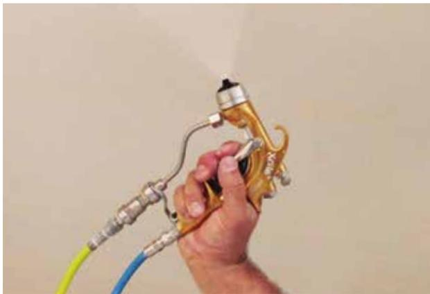
When the final layer of plaster has been applied and the desired finish is achieved, spray the surface with Even Better Acoustical Coating in the chosen color.
