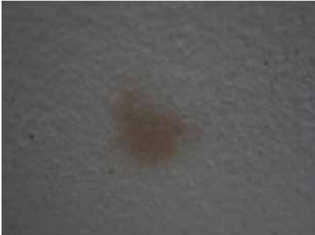
**Resin Spots:** Must be treated by cutting into the affected basecoat and Even Better Acoustical Board to remove the resin deposit. Fill the extracted area with new board, basecoat and sand when dry.
