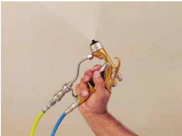
When the final layer of plaster has been applied and the desired finish is achieved, spray the surface with Even Better Acoustical Coating in the chosen color. Ensure the Even Better 2 Silk plaster is fully dry and cured prior to spraying the Acoustical Coating.
