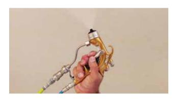
When the final layer of plaster has been applied and the desired finish is acheived, spray the surface with Even Better Acoustical Coating in the chosen color.
