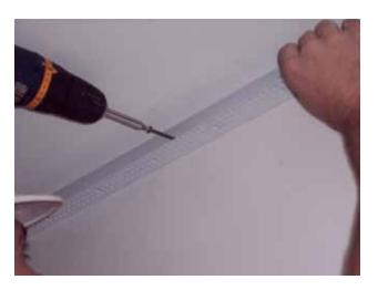
Screw the plastic C channel trim into the perimeter wall 400 mm c/c (16" o.c.) studding and not the ceiling.
