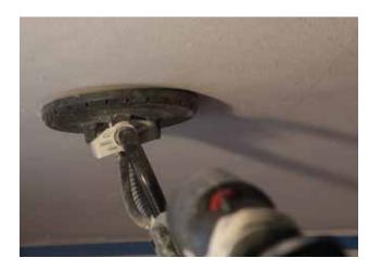
The Silk finish consists of a base layer of Even Better 1 top coat of Even Better 2 plaster and a finish coati of Even Better Acoustical Coating. Sand the base layer application with a 220 grit sanding disc and sanding sponges. Once sanding is complete all imperfections should be eliminated including any board joints, holes, or trim details.
