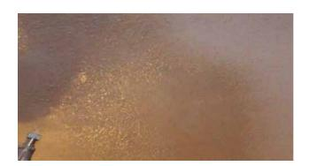
The objective is to spray the Even Better 1 finish onto the basecoat leaving a fine sprayed texture.
