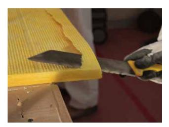
On any boards that will slot into the plastic C channel you need to bevel the edge by trimming the back edge of the fiberglass board as this will enable it ease into the channel; keep these slivers for joint preparation work.
