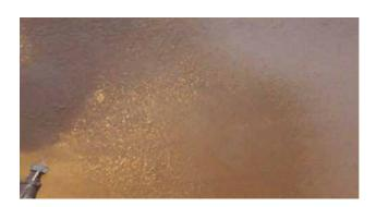
The material flow would normally be set the 3rd ascending dot on the Graco RTX 5000 Pl. Mix up the top coat in the same manner as the basecoat.
