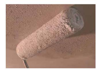
Apply the Alcro Tät Primer mixed with Primer additive to the drywall substrate with a short nap roller.
