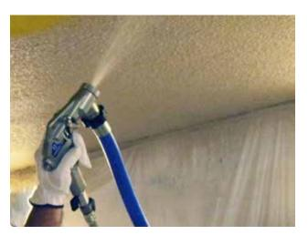
The objective is to spray and trowel the basecoat onto the Even Better Acoustical Board at 3 mm (1/8") wet thickness as the dry thickness will be approx. 1.5 mm (1/16").
