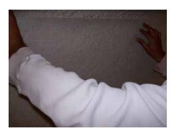
Apply approximately 70% of the basecoat as normal to the surface. Place each vertical length of mesh as you proceed along the length of a wall spraying basecoat. Do not overlap the mesh. Try and butt the lengths as tight as possible. A small gap of 13 mm (1/2") is acceptable.
