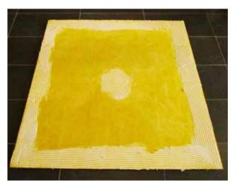
Apply the Even Better Adhesive to the back of the board by using a 6 x 6 mm or 1/4" notched trowel. Make sure to fit the acoustical boards before any coating appears on the adhesive.
