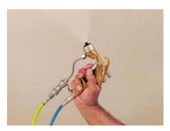
When the final layer of plaster has been applied and the desired finish is acheived, spray the surface with Even Better Acoustical Coating in the chosen color.
