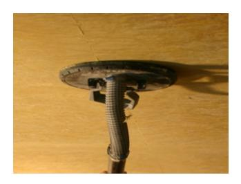
Sand the entire surface of the acoustical board in a gradual circular motion to ensure the board joints are sanded flush and all variances are sanded out. i.e. eliminating valleys, "low points or lines" in the board substrate. Use 80 grit full size sanding disc pads. The completed board installation should appear to be consistent with no variances in thickness. Ensure the critical lighting is in place prior to sanding to ensure any variances are sanded.
