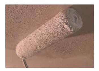
Apply the Even Better Primer mixed with Primer additive to the drywall substrate with a short nap roller.
