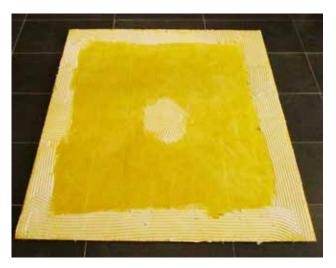
Apply the Even Better Adhesive to the back of the board by using a 6 x 6 mm or 1/4" notched trowel. Ensure to apply the adhesive along all edges of the board and at all ceiling pentration cut outs. Apply a few dots of glue in center of board as well. Press the board and shear it into place. (see picture to the left). Uneven or curved surfaces require more adhesive.
