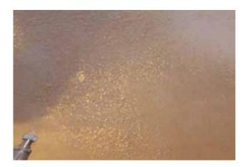
The objective is to spray the Even Better 1 finish onto the basecoat leaving a fine sprayed texture.
