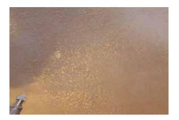
The Silk finish consists of a base layer of Even Better 1 top coat of Even Better 2 plaster and a finish coating of Even Better Acoustical Coating.
