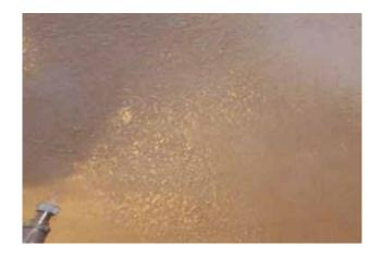
The objective is to spray the Even Better 1 finish onto the basecoat leaving a medium to rough sprayed texture.
