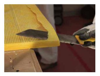
On any boards that will slot into the plastic C channel you need to bevel the edge by trimming the back edge of the acoustical board as this will enable it ease into the channel. Cut as narrow as possible; keep these slivers for joint preparation work.
