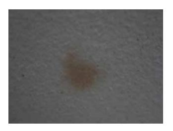
**Resin Spots:** Must be treated by cutting into the affected basecoat and Even Better Acoustical Board to remove the resin deposit. Fill the extracted area with new board, basecoat and sand when dry.
