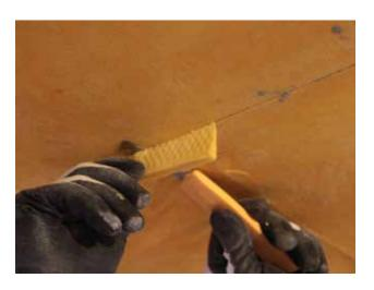
Ensure the spliced material is wedged very tightly into any gap and cut flush in preparation for sanding. You can use the beveled cut shavings from the boards that were inserted into the C channel. It is critical that the boards are installed and prepped correctly.
