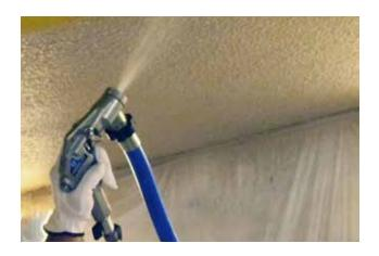
The objective is to spray and trowel the basecoat onto the Even Better Acoustical Board at 3 mm (1/8") wet thickness as the dry thickness will be approx. 1.5 mm (1/16"). 3 mm(1/8") thickness corresponds to just thick enought to eliminate yellow shine through from the board. Tip Size:
