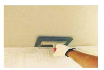
Spray in a small circular motion approximately 3 m2 (30 sqft) and have applicators start to trowel the plaster.
