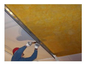
As you progress with the installation of the acoustical boards you may have to periodically "straighten the line" as depicted. The Even Better Acoustical Boards are manufactured to a tolerance of 3 mm (1/8"); therefore, this straightening process is normal.
