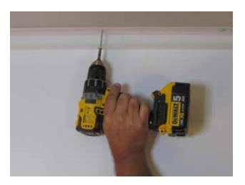
Screw the plastic C channel trim into the ceiling grid studs directly, or through the GWB.
